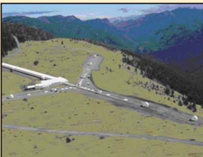
(Above) Artist's impression of the interferometer at the Magdalena Ridge Observatory. The array will consist of up to ten telescopes in a Y configuration, operating in the optical and near-infrared wavelength. Further information can be found on the Magdalena Ridge Observatory website at www.mro.nmt.edu
