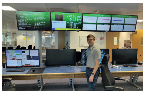
OSL engineer Phil Smith working in the Control Room at Diamond Light Source
